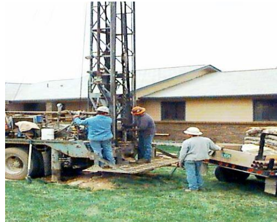
Well construction near Northglenn
